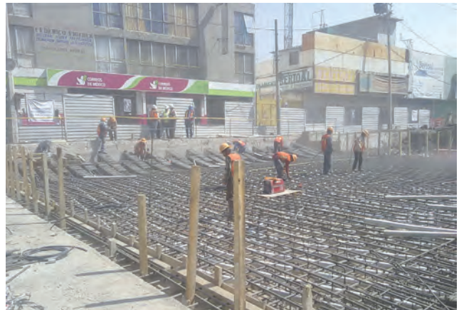
Subway, Mexico City
