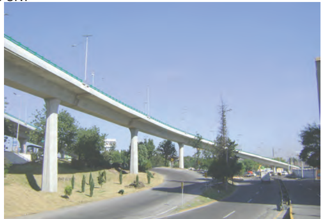
Bicentennial Viaduct, Edo. de México
