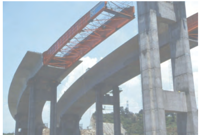
La Marquesa Bridge, México-Toluca Highway.
