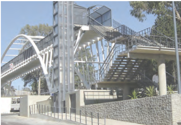
Tlalpan Footbridge, Mexico City
