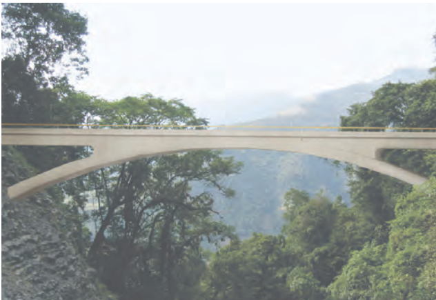
Zoquitlan Bridge, México - Tuxpan Highway
