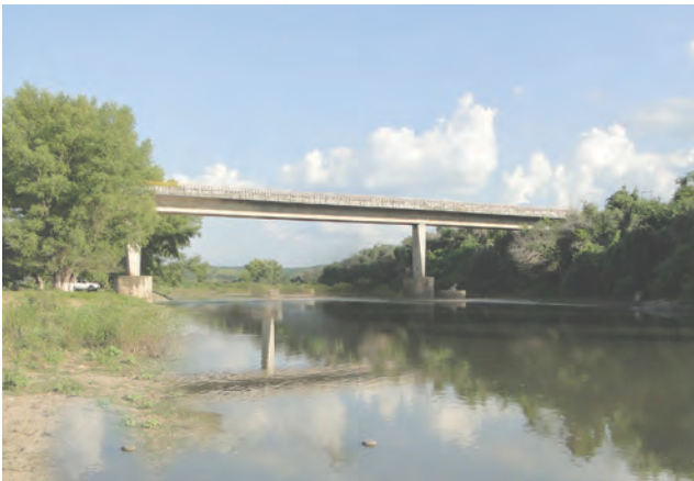
Badiraguato Bridge, Sinaloa, Culiacán.
