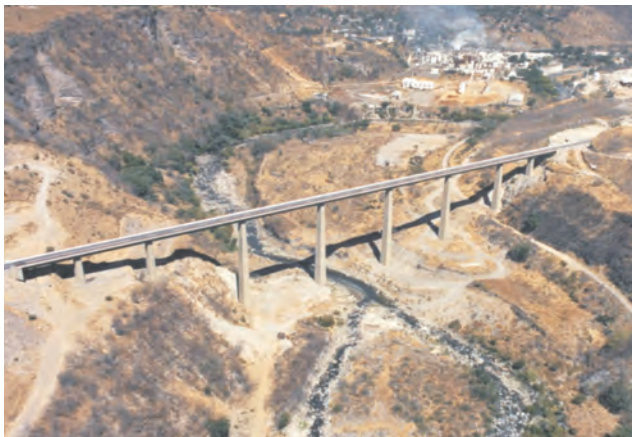
Atenquique II Bridge, Guadalajara-Colima Highway
