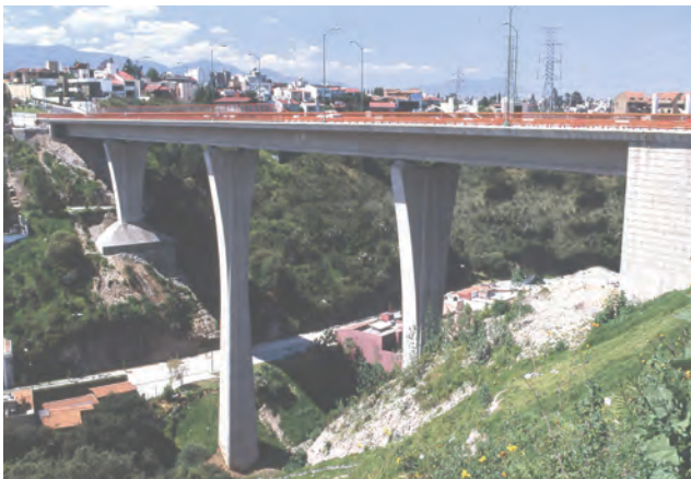
Huixquilucan Bridge, Mexico City
