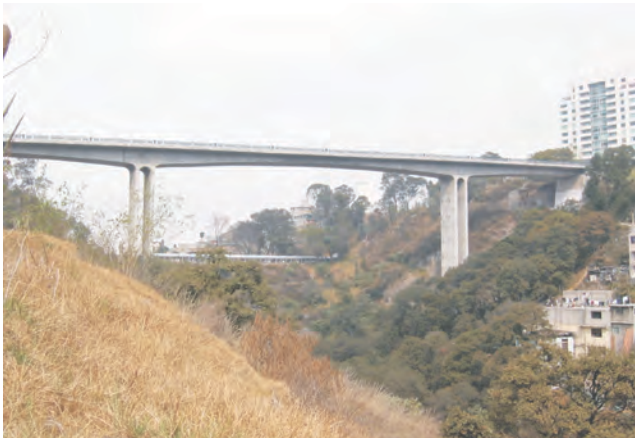
Lomas Country, Bridge, Mexico City
