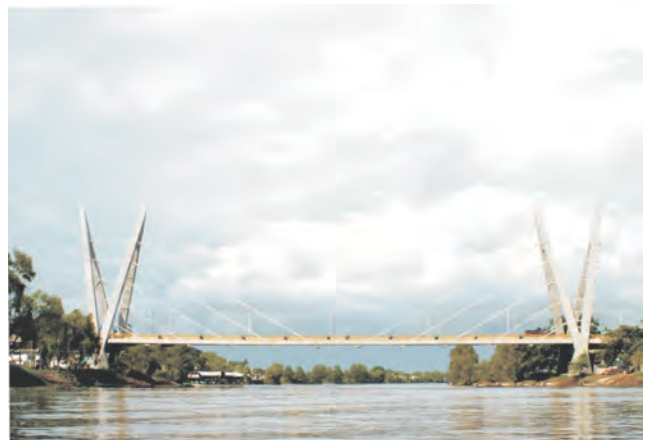
"Grijalva I" Bridge, Villahermosa, Tabasco
