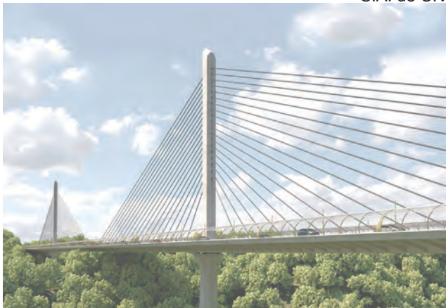
Carrera Novena Viaduct, Bucaramanga, Colombia
