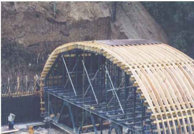
Alcantarilla "Bosque Real", Huixquilucan Edo. Mexico
