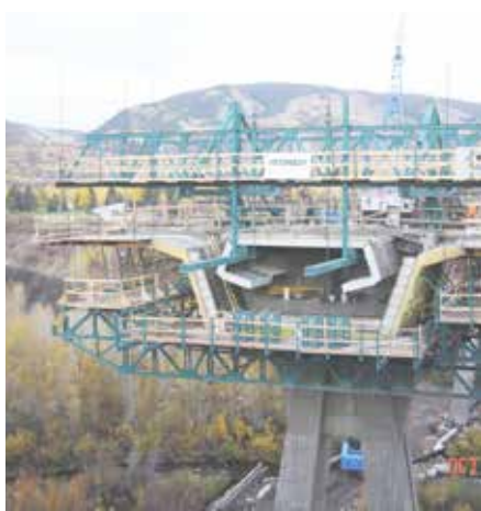
Maroon Creek Bridge, Colorado, USA
